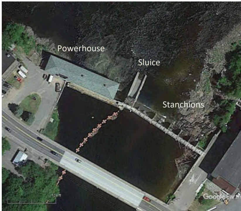
Photo 3. South Dam, powerhouse, downstream sluice and stanchions.
