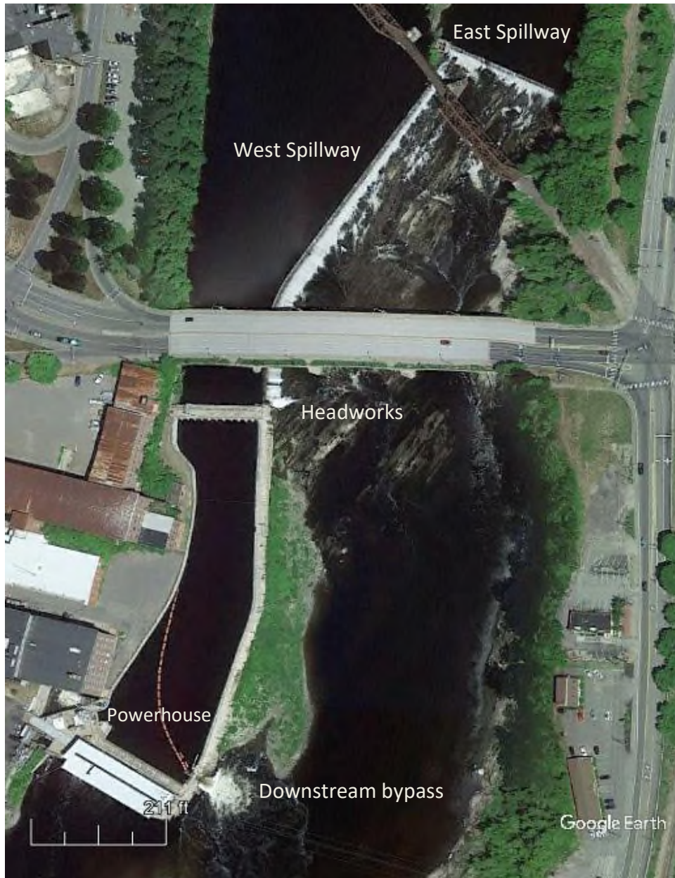
Photo 7. Lockwood Project, east spillway, west spillway, headworks, powerhouse, and downstream bypass.
