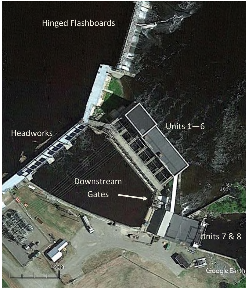
Photo 5. Shawmut powerhouses, downstream bypass gates, headworks, and hinged flashboards.
