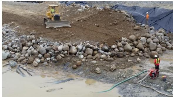
They created conditions resembling a natural stream by forming a series of resting pools and riffles through the low-flow channel, shaping a shallower overbank area, and strategically placing large boulders to generate the desired hydraulics. The result was a structurally stable channel incorporating a diverse set of river features and hydraulics, ready to pass a range of fish species under varying flow conditions.
