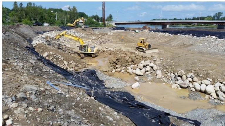
The Howland natural bypass channel design is one of the largest and most complex ever constructed on the East Coast. The bypass is already accommodating a wide range of flows as intended,
