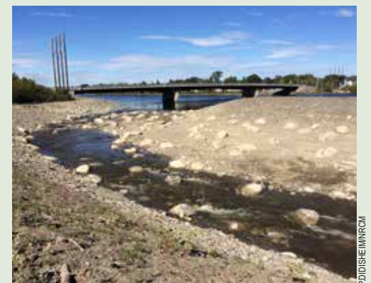
Howland dam bypass construction September 2015
