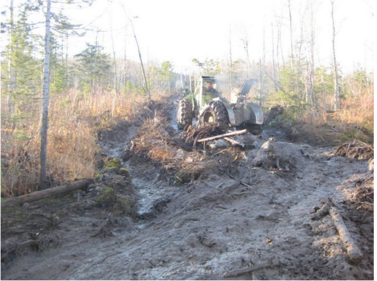
Mud flows.....5 skidders were to work this access road today.
