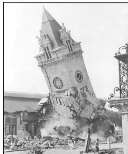
Demolition of Union Station, Portland
