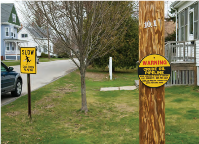
The Portland-Montreal Pipe Line flows underground through dozens of communities throughout New England and central Canada.
