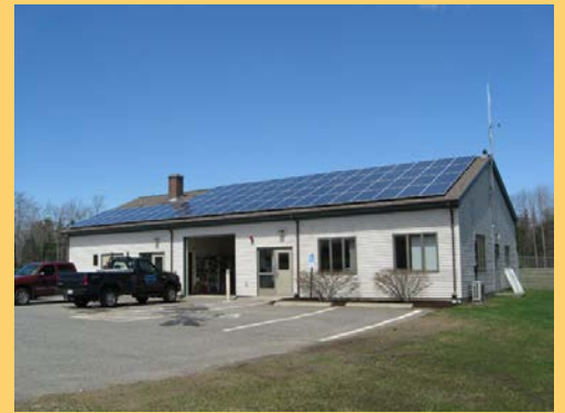
The Town of Thomaston's wastewater treatment plant installed 78 photovoltaic panels on the roof of its building with the help of a rebate from Maine's now expired solar rebate program. The 18 kW solar array generates 13 percent of the plant's heavy electricity needs.
