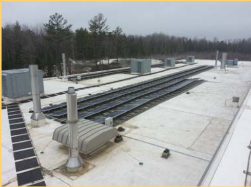
Mt. Blue School in Farmington benefits from a 30 kW solar electric system that will reduce the school's electricity bill for the next 25 years. The solar array is combined with energy efficiency measures that lower costs and increase sustainability.
