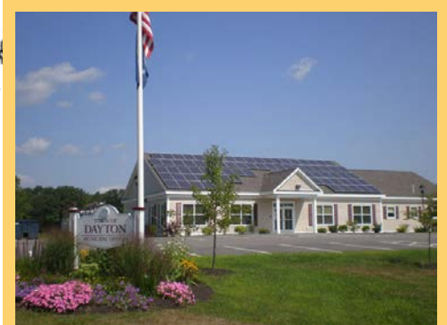
The Town of Dayton's municipal building , with the help of the 15 kW solar power array, enjoys electric bills of nearly zero year-round, saving thousands of dollars annually.
