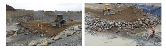
They created conditions resembling a natural stream by forming a series of resting pools and riffles through the low-flow channel, shaping a shallower overbank area, and strategically placing large boulders to generate the desired hydraulics. The result was a structurally stable channel incorporating a diverse set of river features and hydraulics, ready to pass a range of fish species under varying flow conditions.
