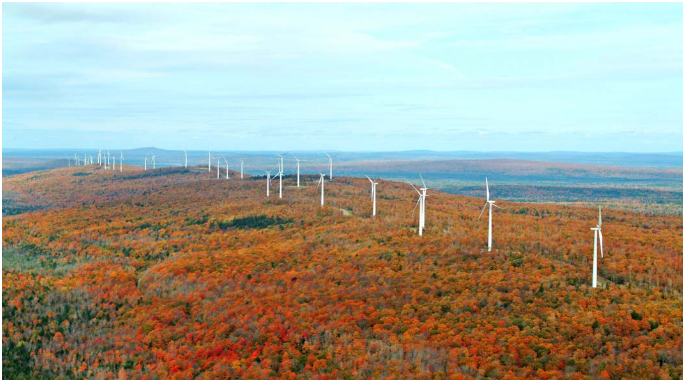
Stetson Wind Farm
