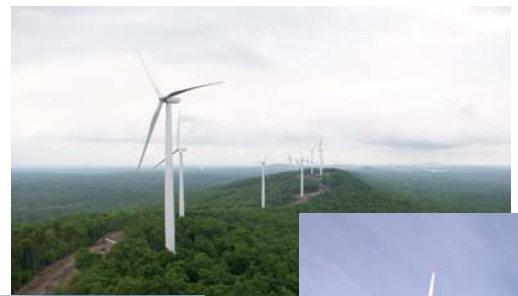
Stetson Wind Farm
