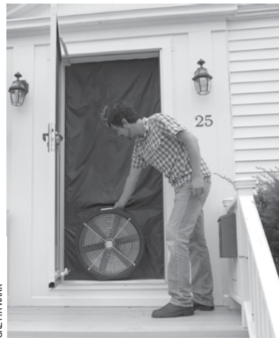
David conducts a "blower test" on Gretta's house to test for energy efficiency.
