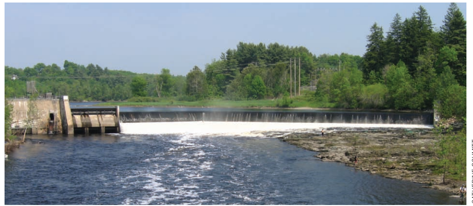
In March, the Town of Winslow Planning Board unanimously approved the removal of the Fort Halifax Dam.
