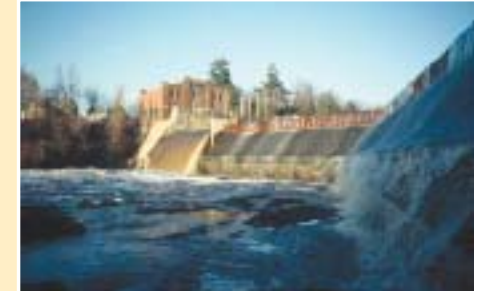
Ft. Halifax Dam
