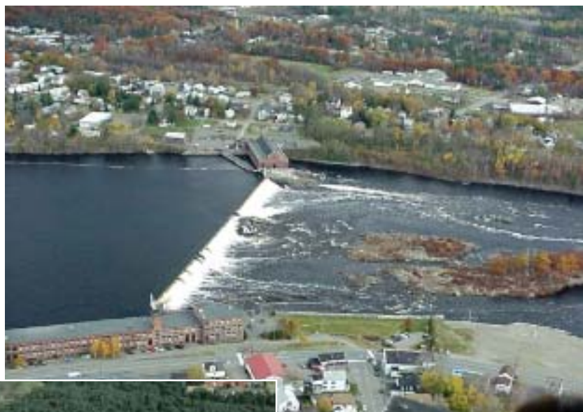
Above: Milford Dam, located between Milford and Old Town on the Penobscot River, has 6.4MW of installed capacity, generating enough electricity for approximately 5,000 households. For reference, Maine has an estimated 518,200 households, according to the 2000 Census.
