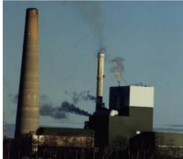
40-year-old Wyman Station in Yarmouth is the State’s largest single source of air pollution because it has not been required to meet modern pollution control standards.
