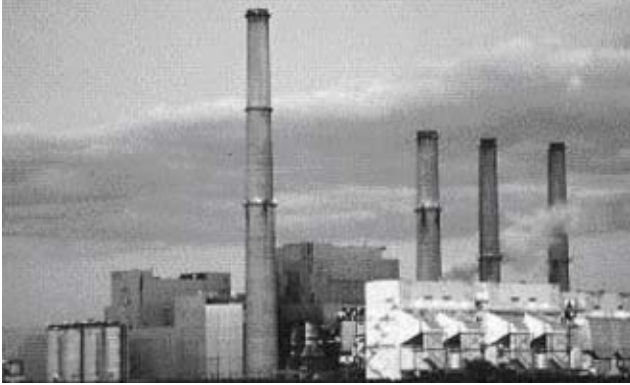
Brayton Point Power Plant in Somerset, Massachusetts is the largest source of air pollution in New England. This 40-year-old facility burns nearly 8,000 tons of coal every day, sending pollution into the air of Rhode Island, Massachusetts, and downwind to New Hampshire and Maine.
