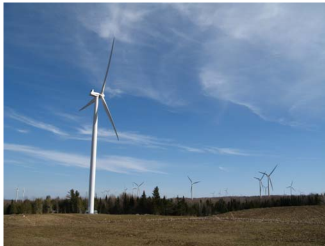
Horizon Wind Energy—Maple Ridge Wind Farm, NY
