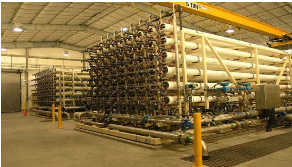
Figure 7: Bingham mine reverse osmosis membranes inside treatment plant
